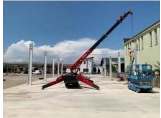
Fig. 1. Small low floor building crane
